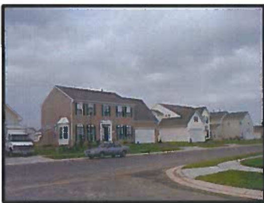
Figure 33: Kent County's housing stock is generally in good condition
