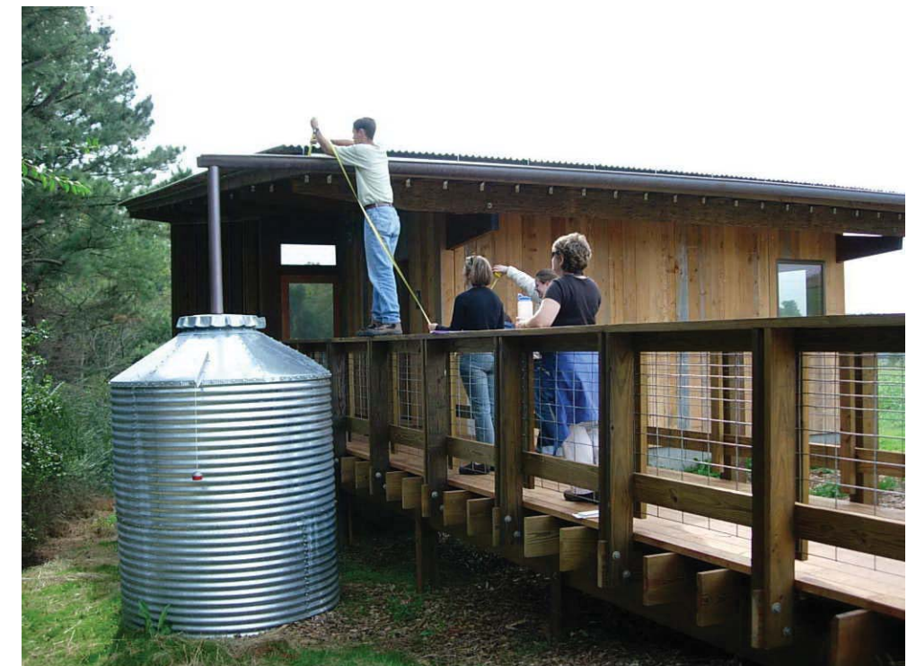
An external cistern is connected to a rooftop provides irrigation water during dry periods.
