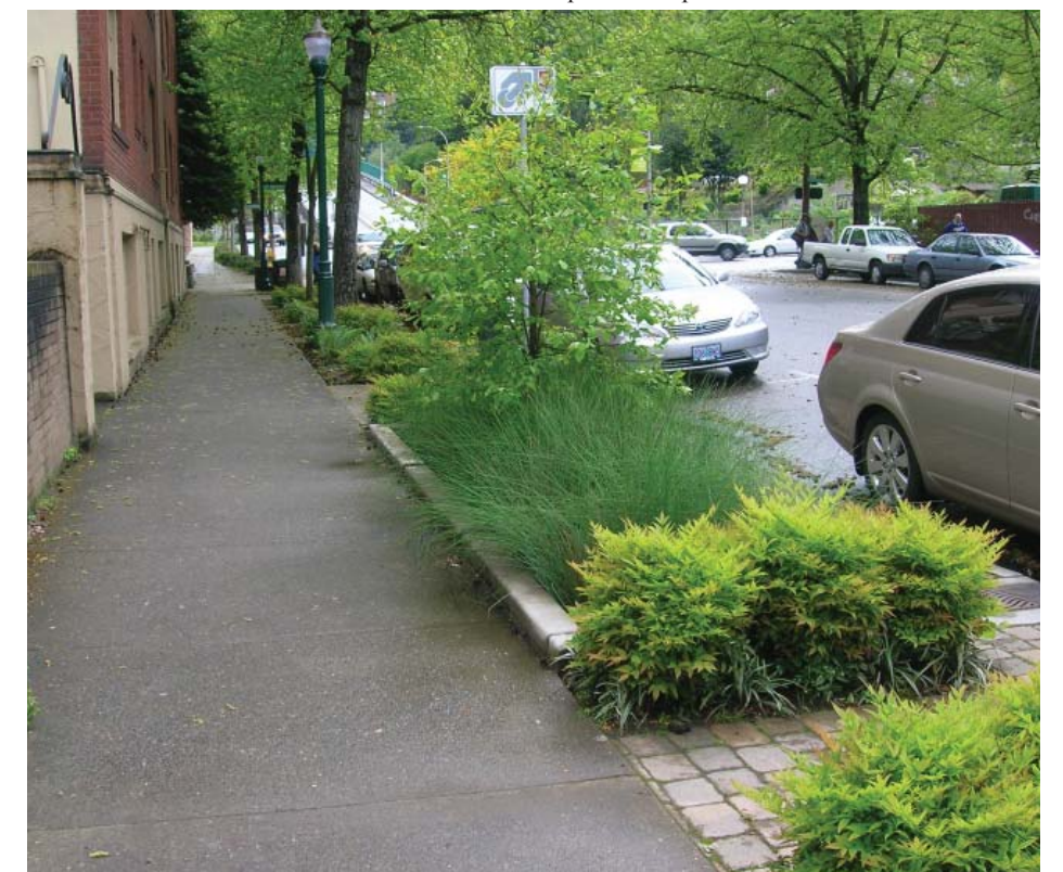
Rainwater run-off receptacle tree planters
