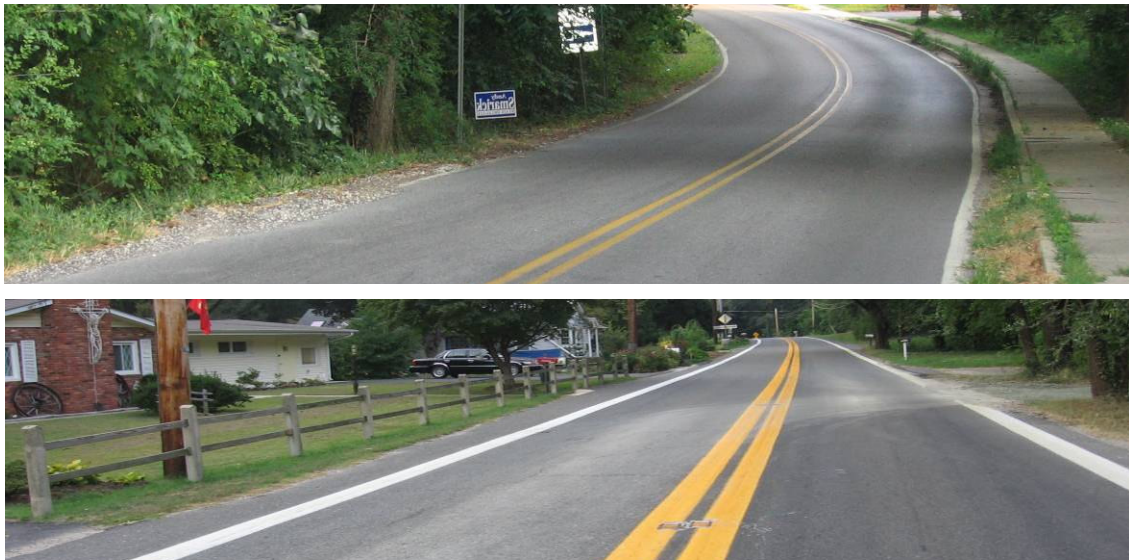
Figure 4-3: Altered pavement striping, such as wider lines, can have noticeable impacts on driver behavior, and is used in many communities. The images above show standard pavement line striping (top) and wide pavement striping on two adjacent roads in Anne Arundel County, MD. Note the width of the centerline and edge lines; the pavement is the same width in both cases.
