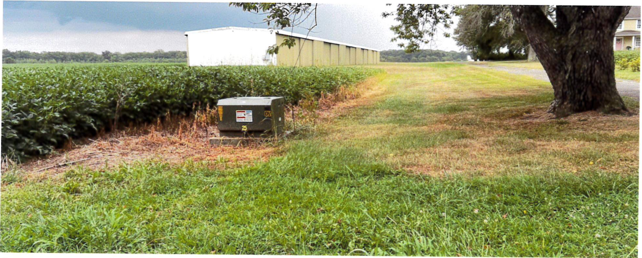
Area on east side of East Driveway (looking due south) where scrubs drown
