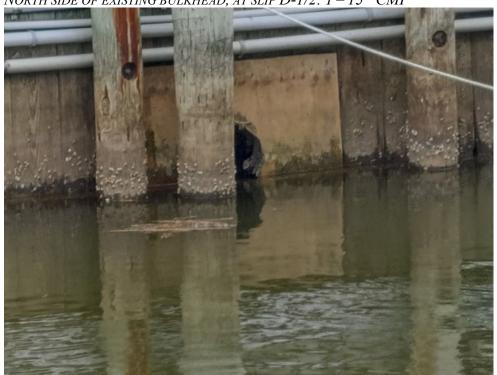
2. EAST SIDE OF EXISTING BULKHEAD, AT SLIP D-9: 1 – 8" PVC, 1 – 18" CMP
