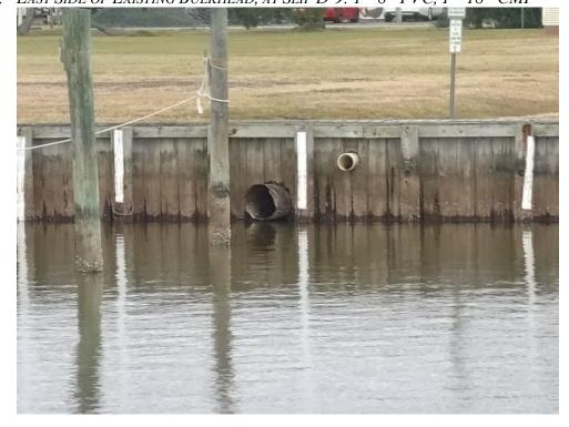
Contractor shall remove a minimum of 8' of existing storm drain pipe. Any existing storm drain pipe removed shall be replaced with an in kind material. Any corrugated metal pipes shall be replaced with BCCMP and appropriate connecting collar / joint.
